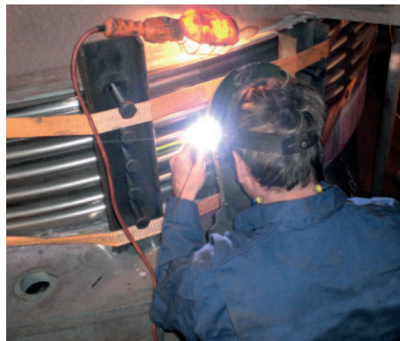
Installation of a clamshell metal expansion joint.
